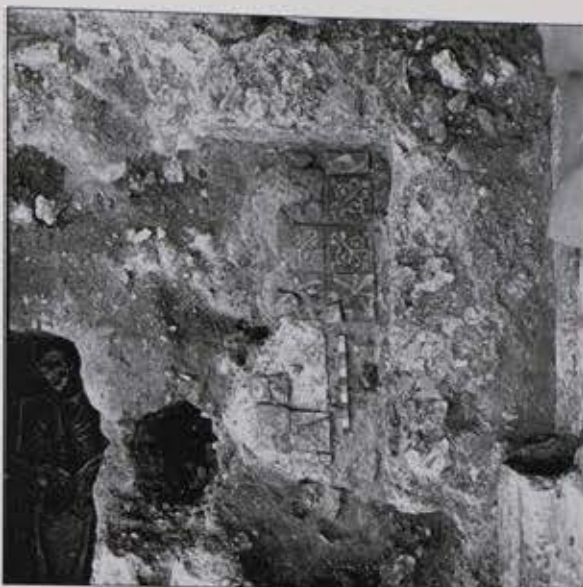
Plate 15. RA 1973: NW corner of the east end chapels. Decorated floor tiles (context 1002) set in the angle of the plinth (context 1091). See Fig 39 (b) for location. (Photograph Kevin Stubbs/TVAT)
