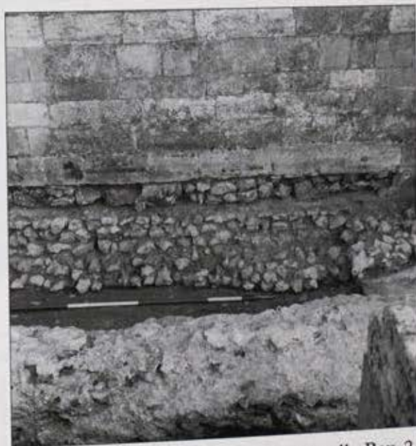
Plate 20. RA 1975: N nave aisle wall, Bay 2, viewed from the N. The Norman flint rubble footing (context 3188=3180) is sealed by a thin mortar layer (context 3081). Above this is the rubble footing (context 3246) of the post-Dissolution blocking of Bay 2. In the foreground is part of the late Saxon north transept. See Fig 27 (a) for location. (Photograph Kevin Stubbs/TVAT)
