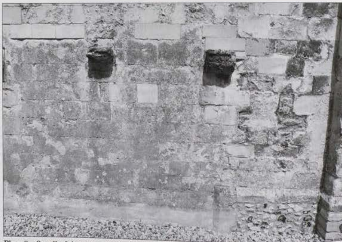
Plate 8. S wall of the nave, detail of bay 4. (Photograph TVAT)
