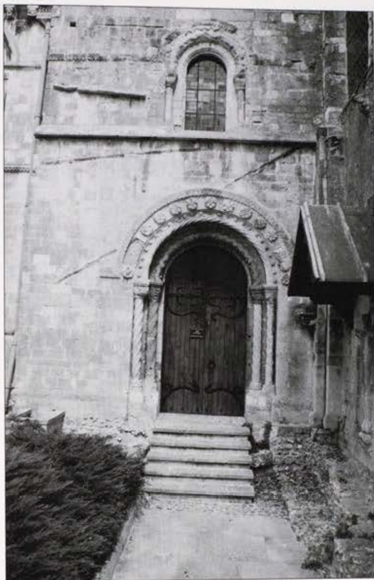
Plate 10. S wall of the nave, showing bay 1 with the Abbess's doorway. Note the evidence for at least three roof lines. The date of the rooflines is uncertain, and some, or all, may belong to the period after the Dissolution. Earlier photographs show the steep lower roofline cutting through the arch over the doorway. The arch has been restored. (Photograph TVAT)
